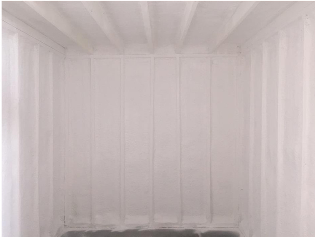
Figure 2. Example of application where the product (white) serves as the thermal barrier over MD spray urethane cavity insulation (and overexposed studs/joists) (1) in wood-frame basement walls and ceiling.
