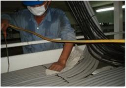
2. Mixing INCA DC6150 cable coating thoroughly by a power agitator before application. Thinner is normally not required. If necessary, use potable water (3% max.) to adjust viscosity. Water is also for
