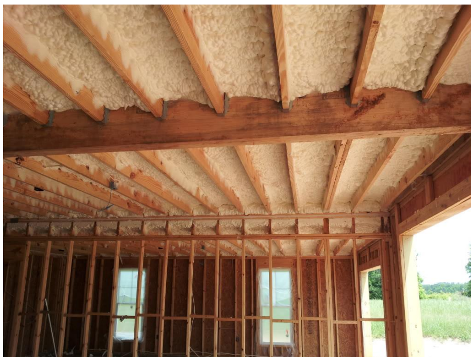
Figure 1. Example of application where DC 315 may serve as a thermal barrier over MD spray urethane ceiling cavity insulation (and joists) 1 within the ceiling of wood-frame garages. (Photo shows spray foam still to be protected with the DC315 thermal
